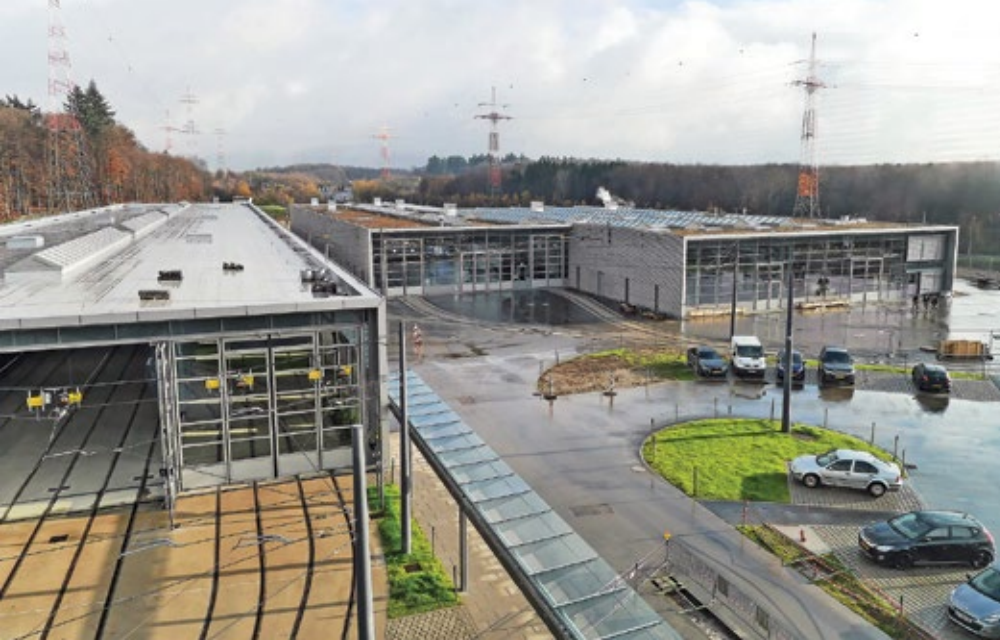
▲ ABOVE: The Tramsschapp , with covered stabling on the left and the main maintenance halls on the right.
