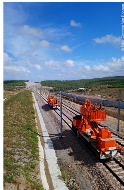
Alongside the civil engineering works, Egis's assignment comprised the programme management for all railway plant and fixtures along the whole of the line (track, catenary, construction depots, etc.). Finally, Egis conducted dynamic testing for track and catenary railway fixtures.
